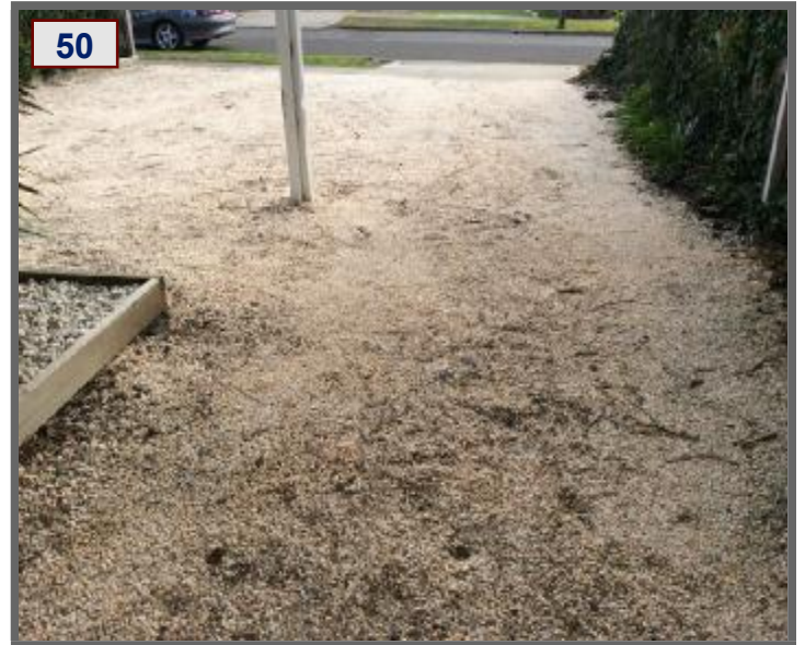
Ungraded Gravel Drive
