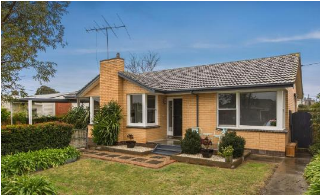
Front Elevation of the Inspected Property
