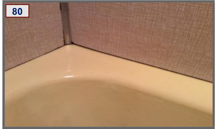
Sealant Around Bath
