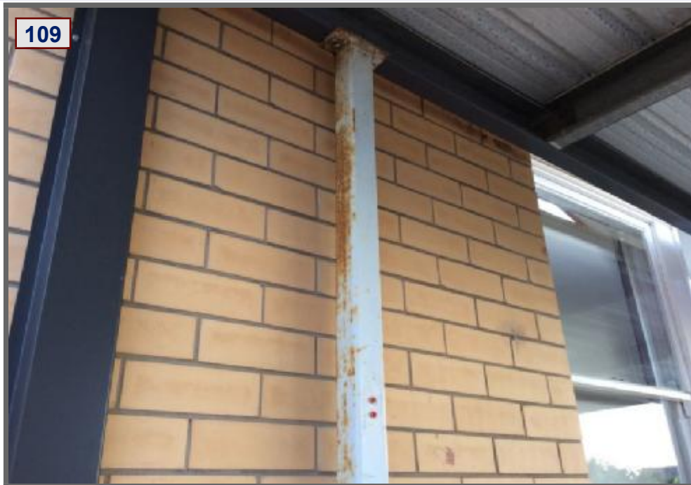
Posts Corroded
