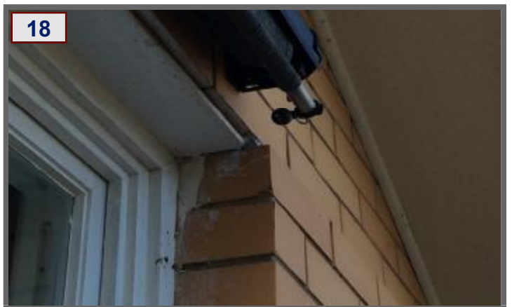
Brick Walls Moved
