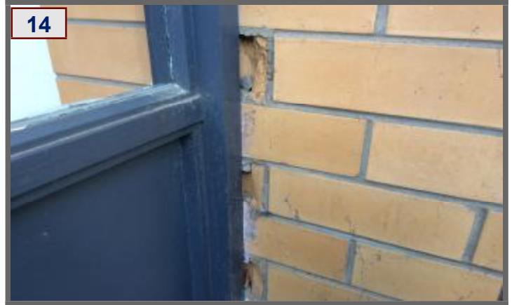
Bricks Damaged
