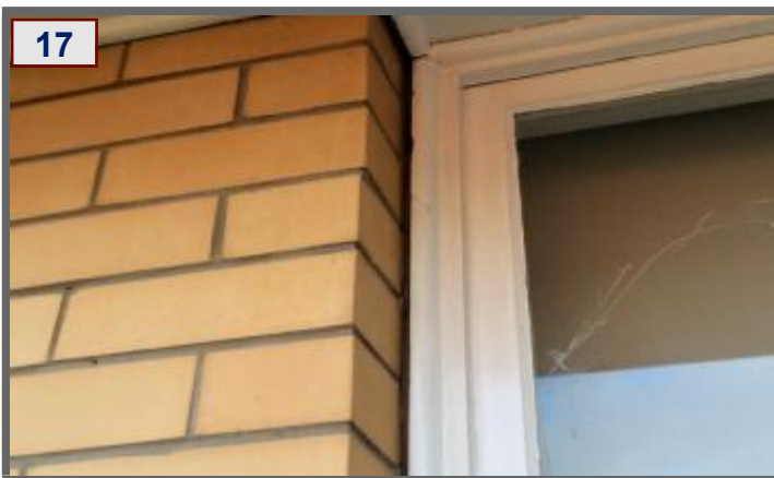
Brick Walls Moved
