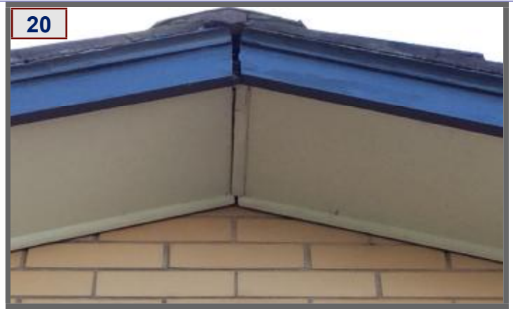
Roof Structure Moved
