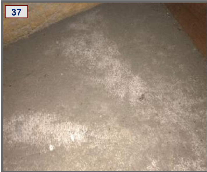
Cement Sheet Ceiling Lining
