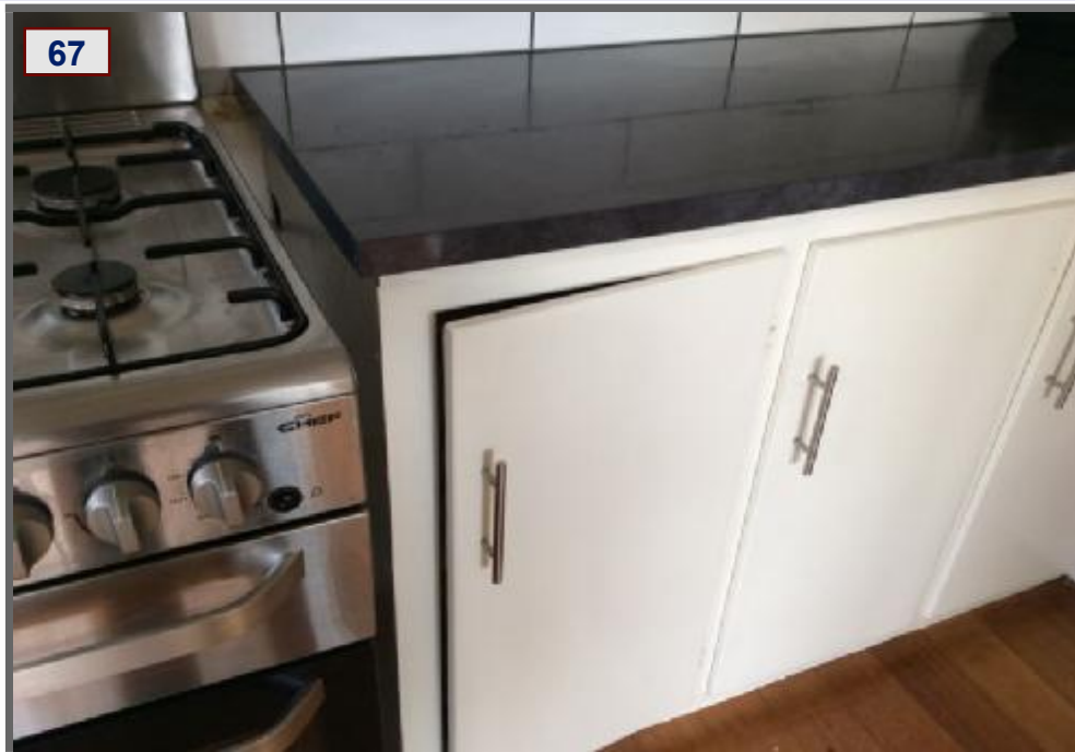
Doors And Drawers Out Of Alignment
