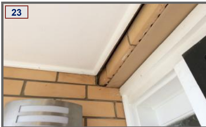
Brick Walls Moved
